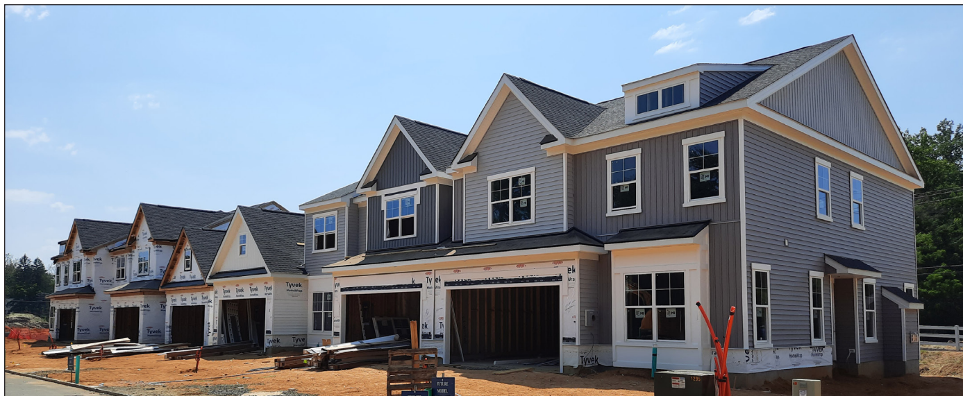
Above: This 30-unit inclusionary housing development in Medford Township, Burlington County, includes 25 market rate units and five affordable housing units. It is being built with the use of 1.75 PDCs, which were redeemed in September 2022.
